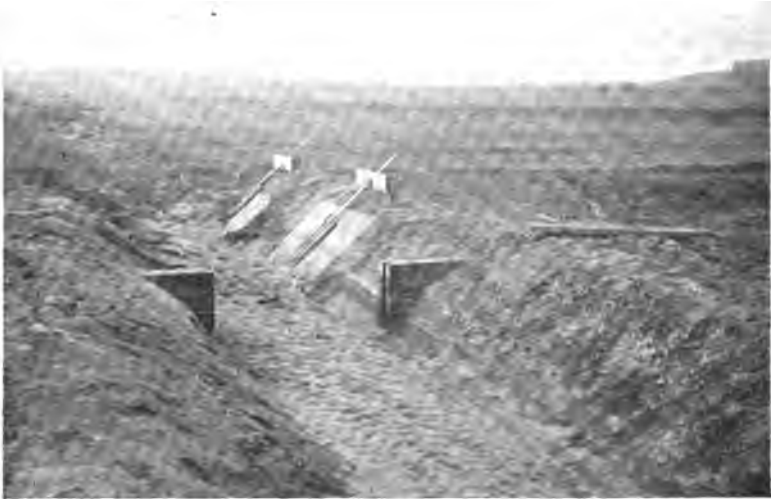
FIG. 104.—Check and Farm Turnout with Inclined Valve.
